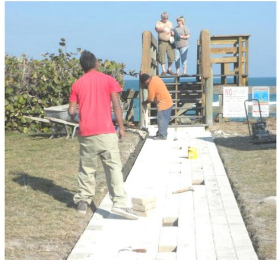
Surfside Pavers of West Melbourne installs pavers for the replacement walkway to the Tampa Avenue dune crossover.
