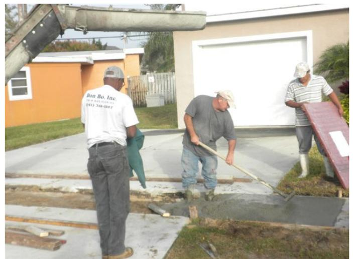
Don Bo, Inc. of Palm Bay recently replaced broken sidewalk along Fourth Avenue. Sections of sidewalk along N. Palm Avenue between Wayne Avenue and Watson Drive and along N. Ramona Avenue were also replaced.
