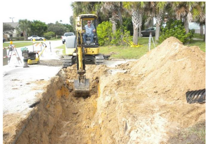
Storm drain pipe under N. Shannon Avenue north of Third Avenue failed and was replaced by Atlantic Development of Cocoa at a cost of \$15,758
