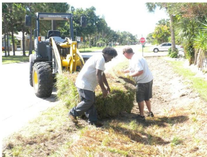
Public Works personnel John Howard and Isaiah Cepeda lay sod at a newly constructed drainage swale along the west side of N. Ramona Avenue immediately north of Michigan Avenue. The swale is part of the Town’s ongoing effort to treat pollution by reducing stormwater runoff. If you would like a swale contact Public Works Director Ron Cassedy at 321-984-5224.
