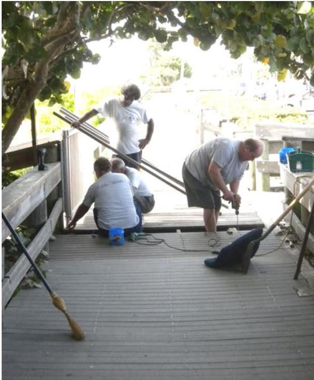
New decking material has been installed on the boardwalk over the past few weeks with all material costs being covered by revenue from the annual Witch Way 5k events and the sale of pavers. Public Works personnel have replaced the ten year old wood deck with TREX material.
