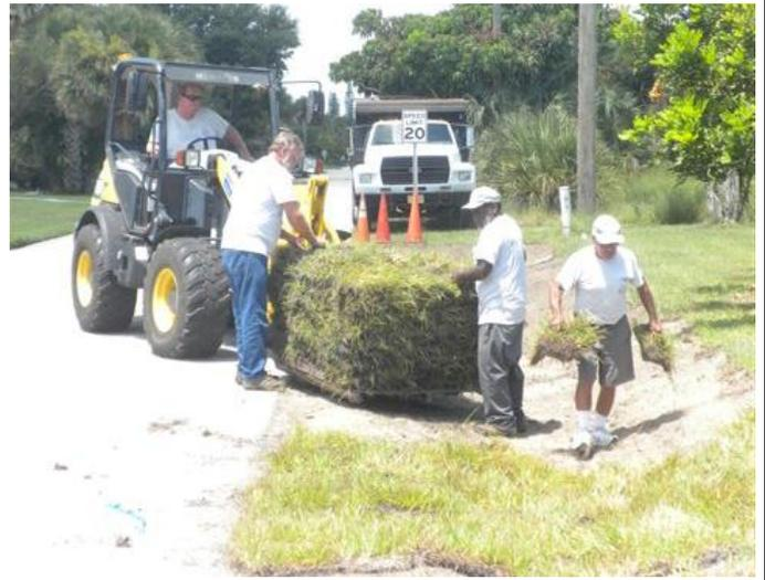
Public Works personnel lay sod at a newly constructed drainage swale along the north side of Wayne Avenue immediately west of Shannon Avenue. The swale is part of the Town’s ongoing effort to treat pollution by reducing stormwater runoff. If you would like a swale contact Public Works Director Ron Cassedy at 984-5224.
