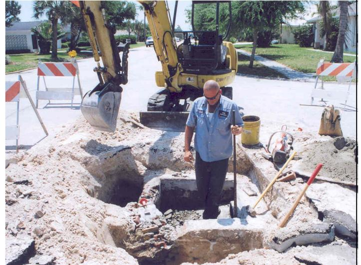
Atlantic Development of Cocoa replaced a failed concrete manhole top on S. Shannon Avenue at Tradewinds Terrace. They also patched a hole that appeared outside of the pavement area
