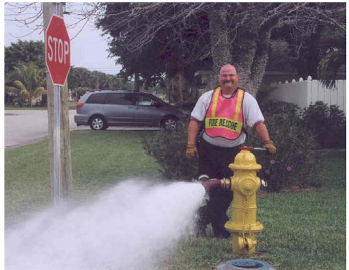
*Firefighter Dave Murtha tests a fire hydrant to ensure that there is sufficient flow and that all of the fittings work should the hydrant be needed. All 86 hydrants in Town are annually tested with deficiencies reported to Melbourne Water*
