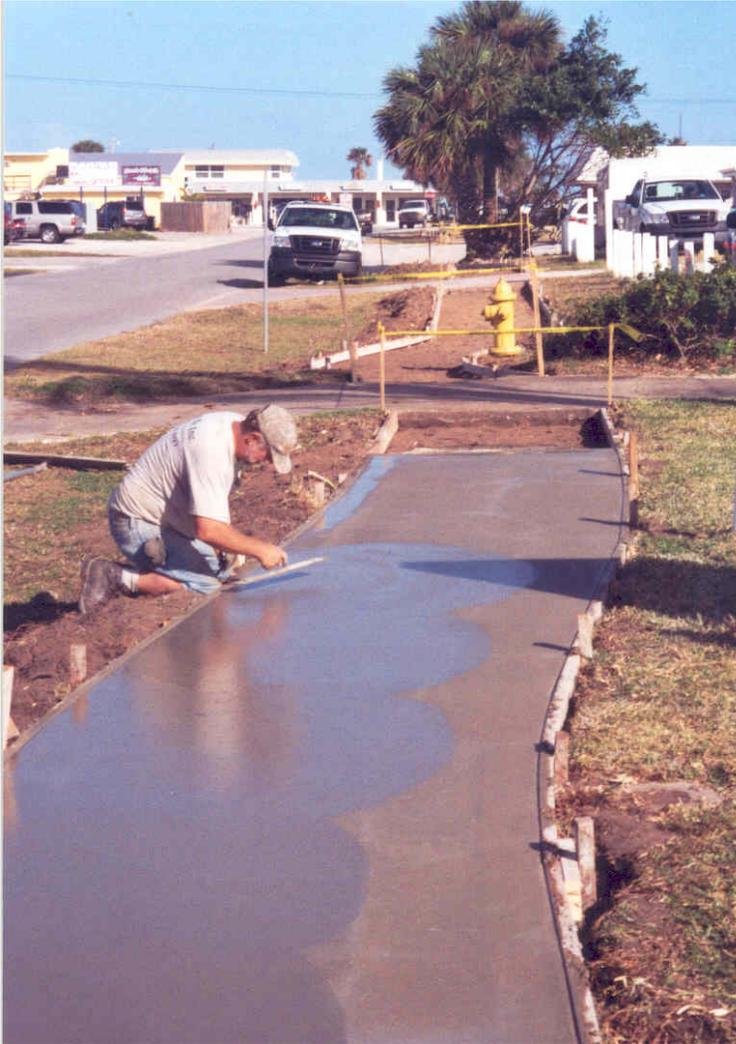
Don Bo, Inc. of Palm Bay completes construction of a sidewalk along the south side of Sixth Avenue in the one hundred block. Three hundred and fifty linear feet of sidewalk connecting the existing sidewalks from S. Miramar Avenue to S. Shannon Avenue was poured in late December and early January.
