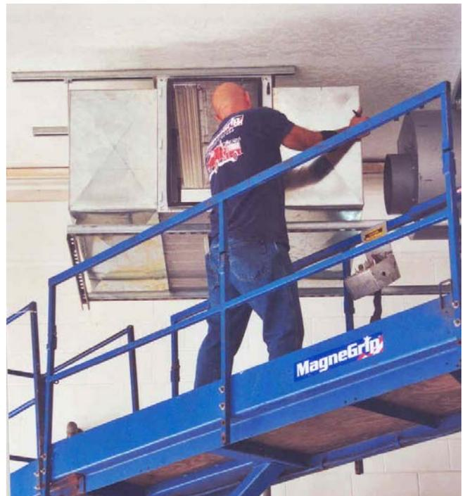
***A Clean Air Concepts representative installs the new exhaust system in the bay portion of the Town's fire station. The system is designed to remove gases and particulates from the station. Funding was provided through a FEMA grant for 95% of the cost with the Town providing the remaining 5% of the \$40,850 project cost. Congressman Dave Weldon presented a ceremonial check representing the Firefighter Assistance grant award in March, 2008.***
