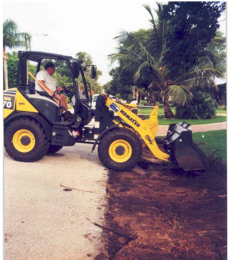
John Howard, with the Public Works Department, constructs a swale at 310 Miami Avenue. Swales are a commonly used stormwater practice recommended to treat runoff to reduce pollution. Property owners desiring to have a swale installed in the street right-of-way in front of their property should contact Public Works Director Ron Cassedy at 984-5224.
