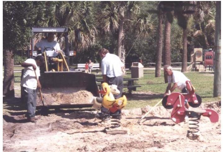
*Public Works personnel remove sand from around Orlando Park play equipment and install FIBAR, which is an engineered wood fiber designed to cushion falls and enable wheelchairs to travel over the area.*
