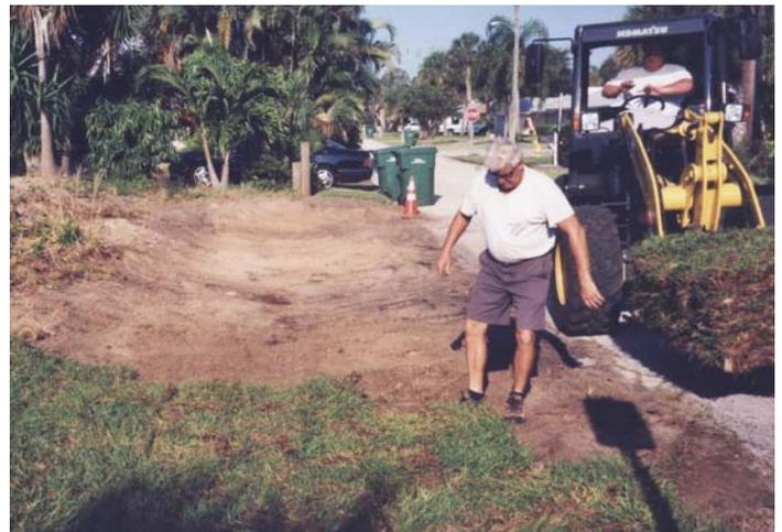
Public Works personnel lay sod after forming a swale in the street right-of-way east of 241 Third Avenue. Swales are a commonly used stormwater practice recommended by federal and state officials to treat runoff to reduce pollution.
