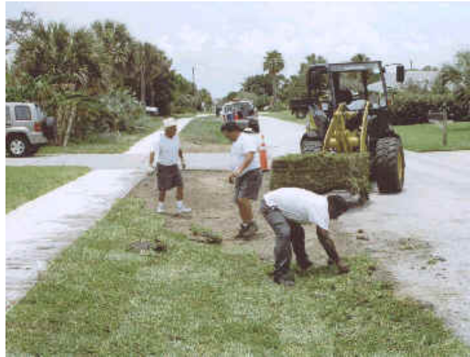
Public Works personnel install a swale at 125 Eighth Avenue
