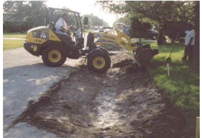
Public Works personnel construct a swale at 429 Eighth Avenue. Swales are a commonly used stormwater practice recommended by federal and state officials to treat runoff to reduce pollutants.
