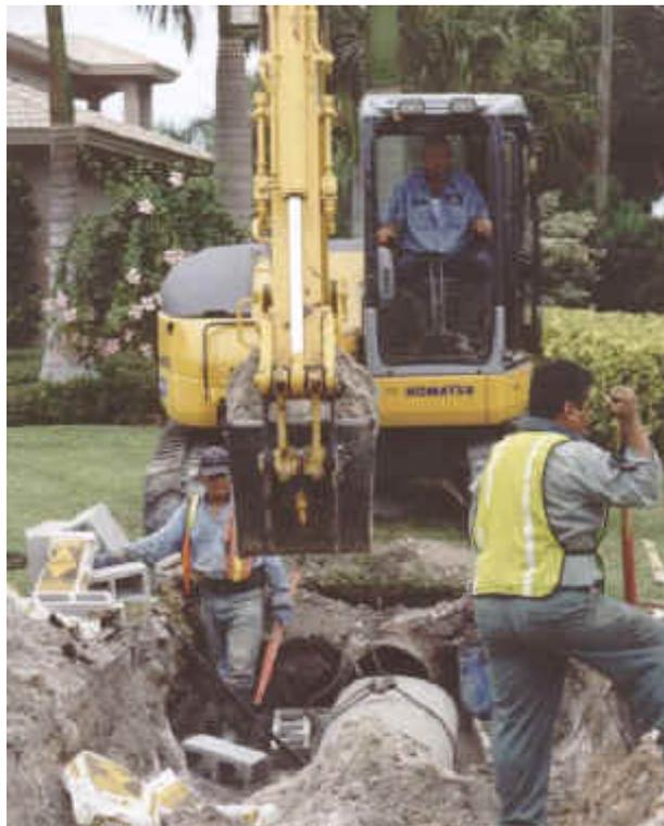
*Atlantic Development of Cocoa, Inc. replaces the failing metal stormwater pipe at 1105 S. Riverside Dr. The Town has approximately 38,000 linear feet of 45 year old metal pipe that needs to be replaced.*
