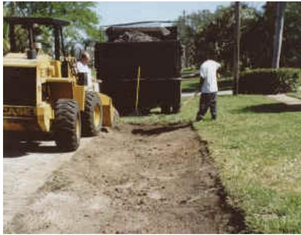
Public Works personnel install a swale in front of 325 Miami Avenue. Council adopted the shallow swale concept in 1991 when it accepted the Stormwater Drainage Report. Property owners desiring to have a swale installed in the street right-of-way in front of their property can contact Public Works Director Ron Cassedy at 984-5224
