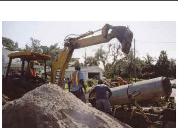
*Atlantic Development of Cocoa, Inc. replaces the failing metal stormwater pipe under S. Riverside Drive at Orlando Boulevard. The Town has approximately 38,000 linear feet of 45 year old metal pipe in need of replacement.*
