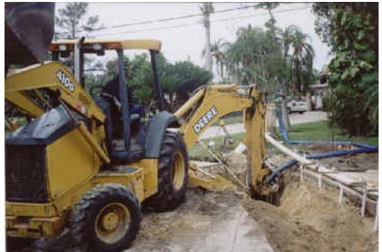
Atlantic Development, Inc. of Cocoa replaces the deteriorated metal drainage pipe under S. Riverside Drive between Melbourne and Eighth avenues
